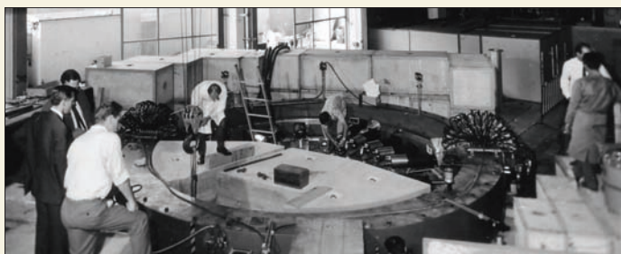
The muon storage ring at the end of the South hall, photographed during installation of the electron counters (inside the ring on the far side) and before the shielding roof was put into place.
