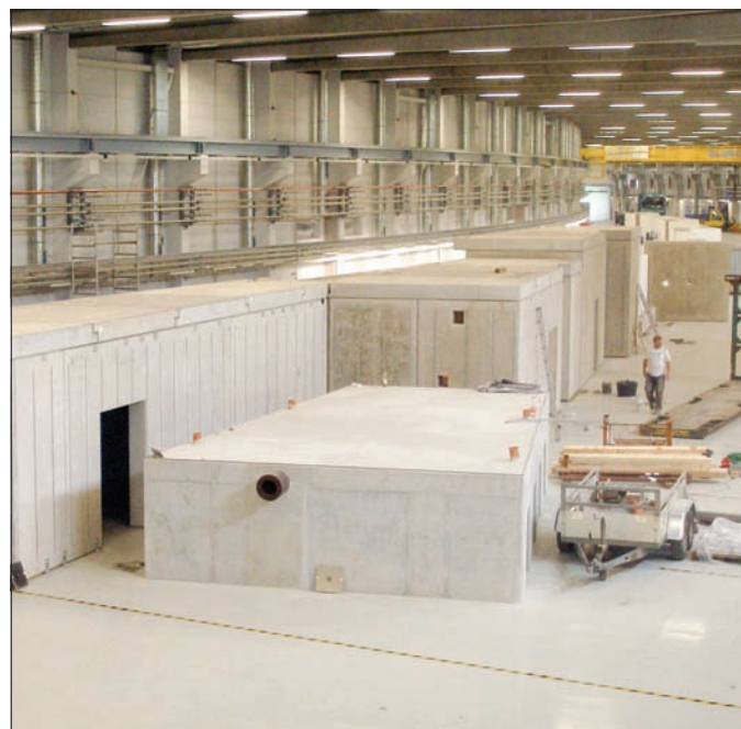
View of the experimental hall. The first optical enclosures are being set up in front of the storage ring tunnel, which is within the white shielding.
